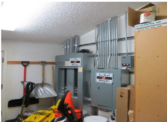
Picture 4 – Main Switchboard Located in Elec. Rm.
