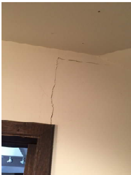
Distress over attic door (north side)
