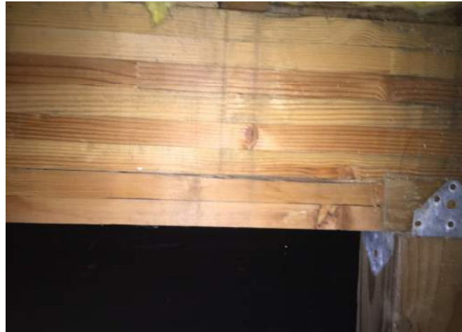
Delamination at the bottom of one glue-laminated beam
