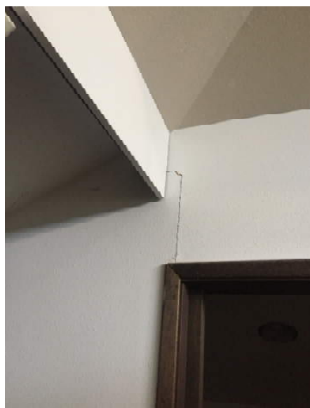
Distress over attic door (south side)
