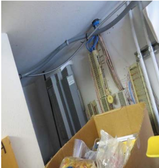
Picture 10 – Main Telephone Terminal Board
