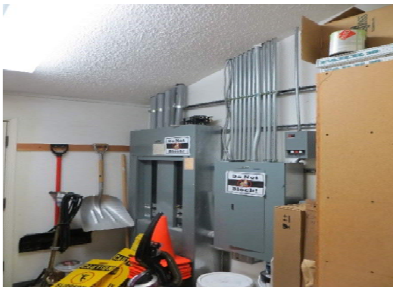
Picture 4 – Main Switchboard Located in Elec. Rm.
