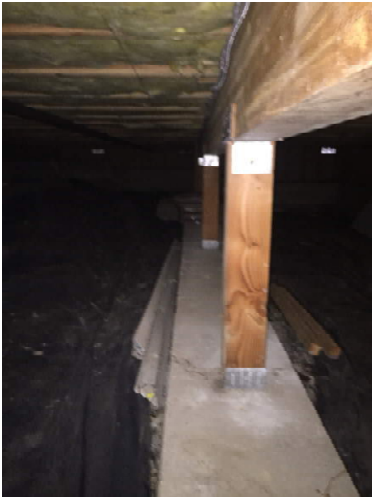
Continuous grade beam in lieu of stem wall & strip footing.
