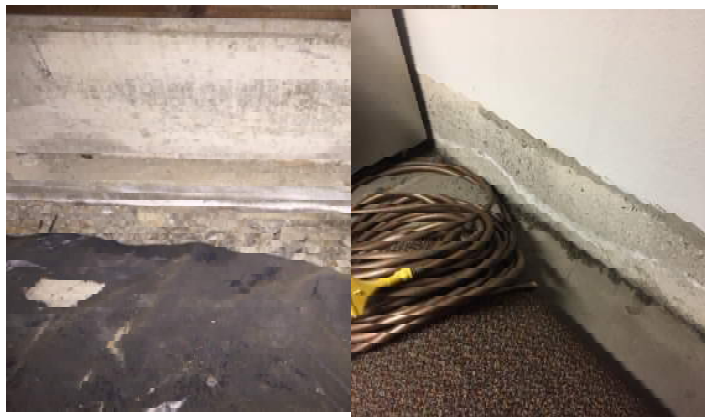
Efflorescence on interior face of exterior concrete construction.
