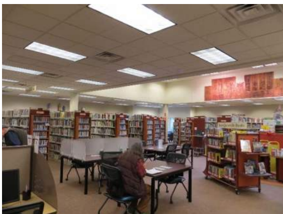
Picture 6 – Existing T8 Fluorescent Lighting
